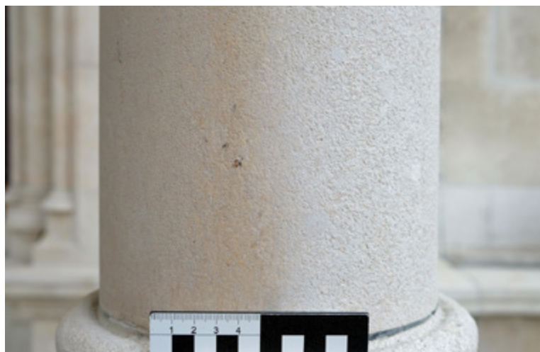
Fig. 4. Detail of a column at the loggia, 2022
